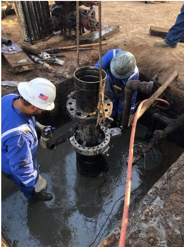
Workers plug and abandon oil wells associated with the Rincon Island Limited Partnership bankruptcy. STATE LANDS COMMISSION
